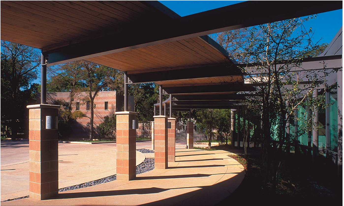
covered walkway to classroom building with Priest's residence beyond
